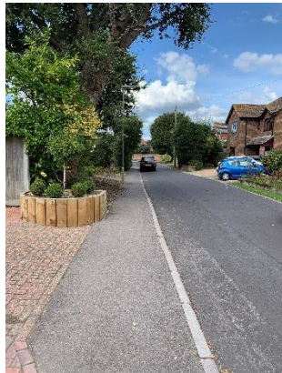
Photograph 47: Conditions on Vicarage Lane
