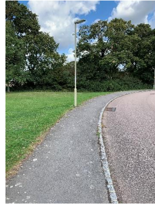
Photograph 26: Marks Tey Road Conditions
