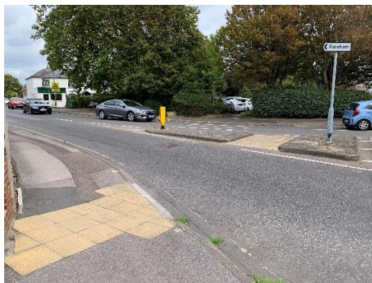
Photograph 20: Pedestrian Refuge Island Crossing at Titchfield Road/May's Lane/Gosport Road Roundabout
