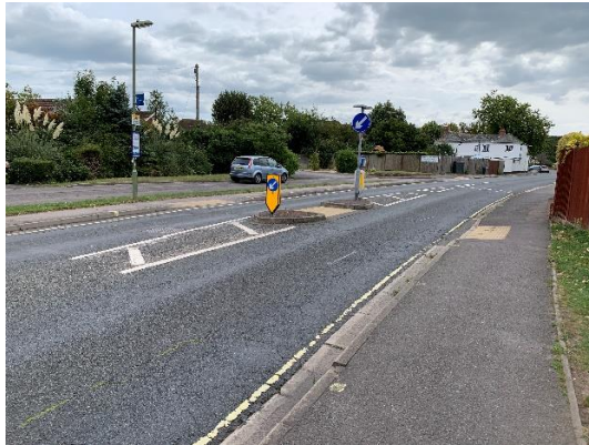
Photograph 18: Pedestrian Refuge Island Crossing 150m north of Titchfield Road/May's Lane/Gosport Road Roundabout
