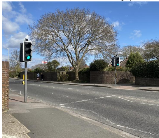
Photograph 57: Signalised Crossing Proximity of Stubbington Green Roundabout
