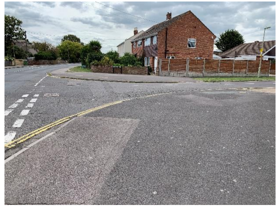
Photograph 15: Green Road/May's Lane Junction
