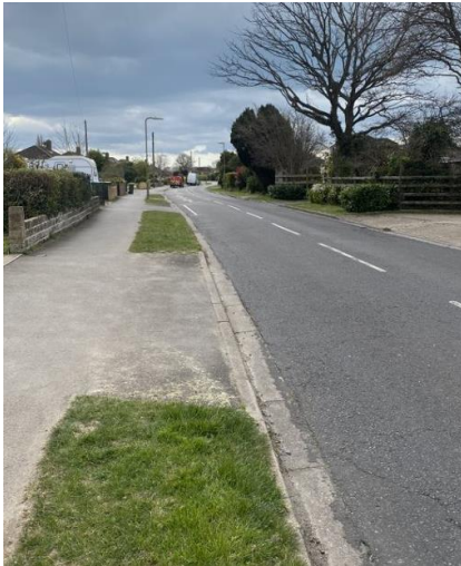
Photograph 37: Conditions on Cuckoo Lane
