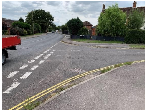
Photograph 16: The Croft/May's Lane junction
