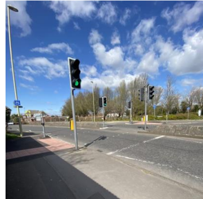
Photograph 22: Signalised Crossing on Gosport Road
