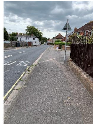
Photograph 19: Conditions on May's Lane
