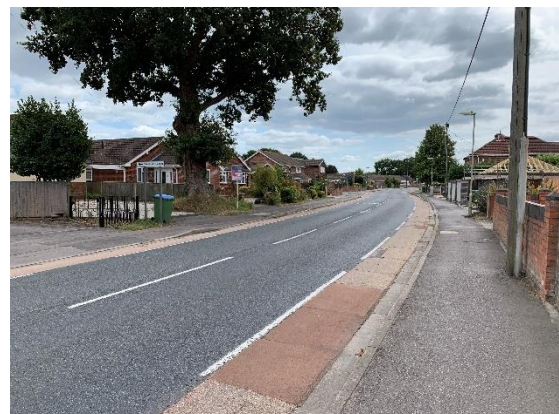
Photograph 13: Conditions on May's Lane
